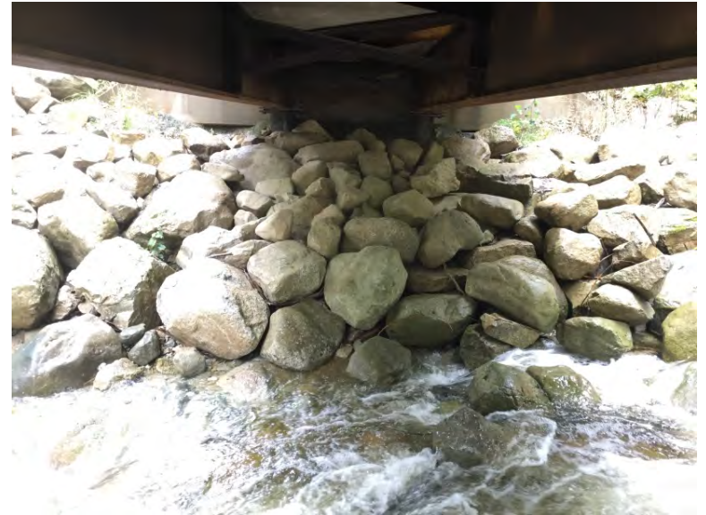
Right Bank Abutment when facing downstream
