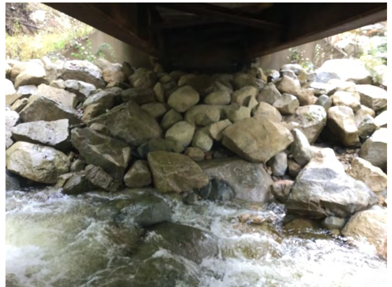
Left Bank Abutment when facing downstream
