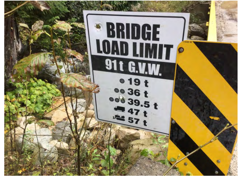
Load Rating Sign
