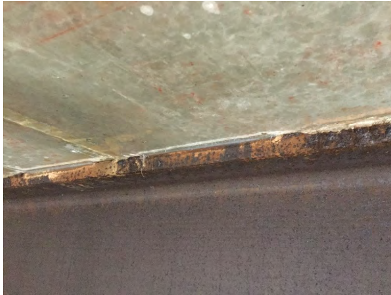
Silicone between deck and girder
